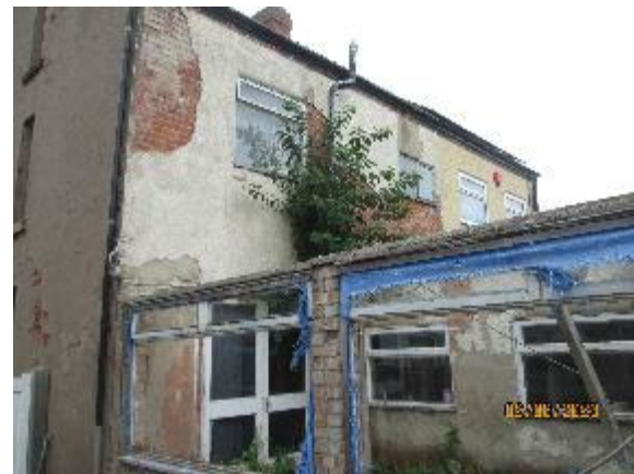
Rear elevation – some elements to be demolished
